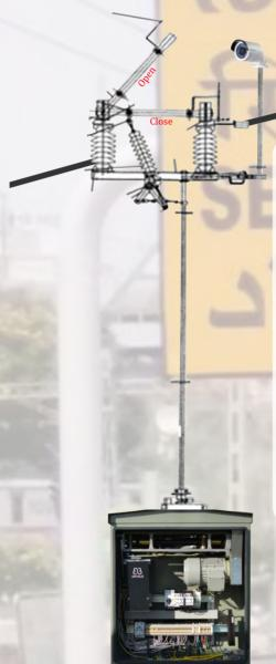
25 KV isolators are needed on OHE to disconnect and earth a section of OHE in loco sheds, washing lines and private sidings so that people can work near the wires. There is a complex safety procedure involved where TPC grants permission to work after proper isolation and earthing.
